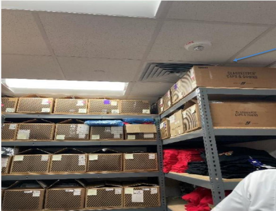
Storage stacked too high. There should be 18 inch clearance from sprinkler heads.
