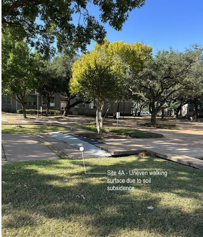
Site 4A - Uneven walking surface due to soil subsidence
